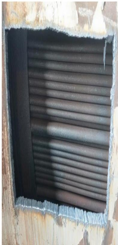
Fig.12: Feed water Heater Tube Bundles
