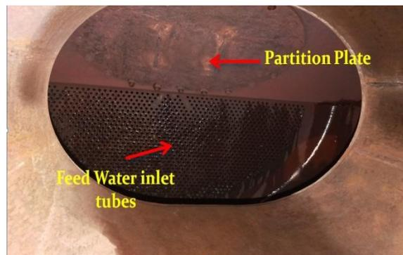
Fig.6: View of water tubes in heater
