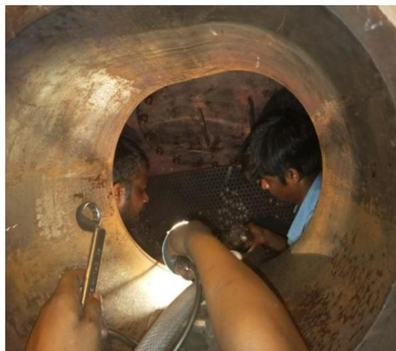
Fig.10: Plugging of tubes
