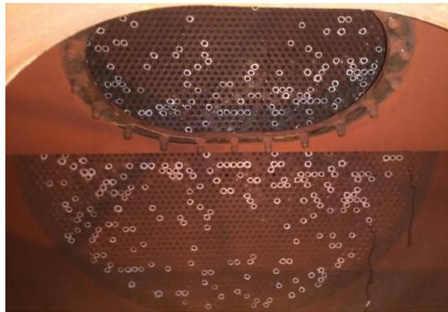
Fig.9: Identified punctured tubes
