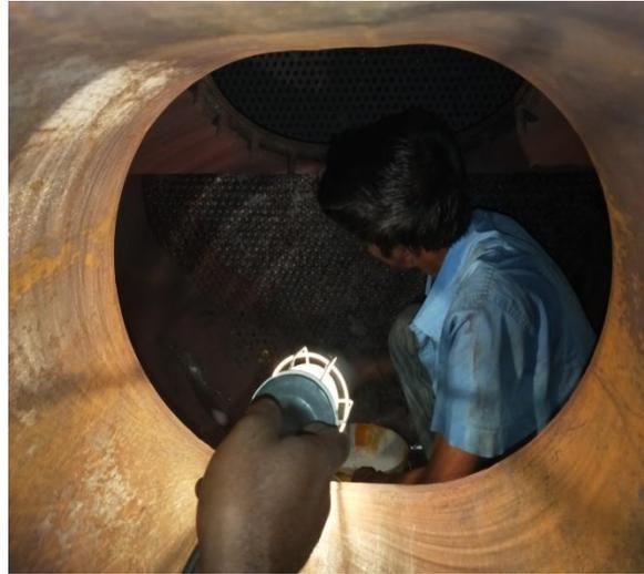
Fig.8: Inspection of Water tubes
