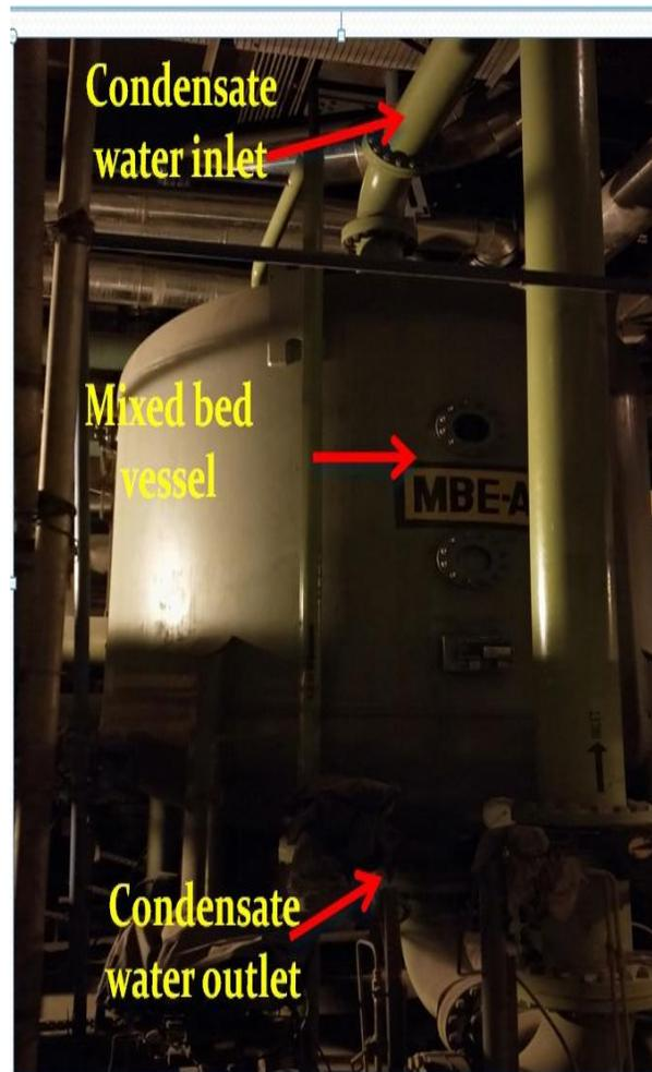
Fig.16: Mixed bed Condensate polishing Unit
