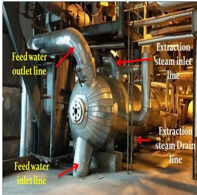
Fig.3: High pressure feed water heater
