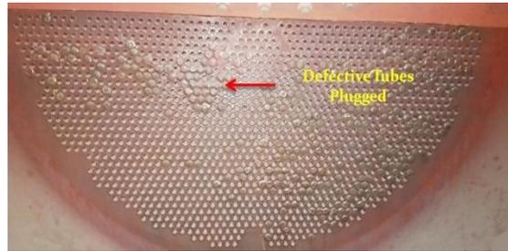
Fig.11: Rectified Feed water tubes
