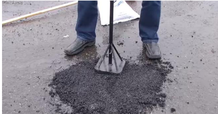
Figure 6.7- Filling Pothole
