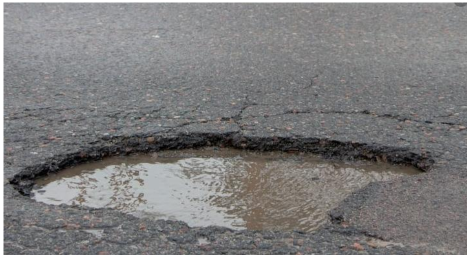
Figure 1.1:Pothole on Road
