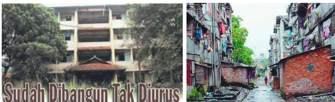
Figure 3: Vertical Housing Problems in Bali, Indonesia
